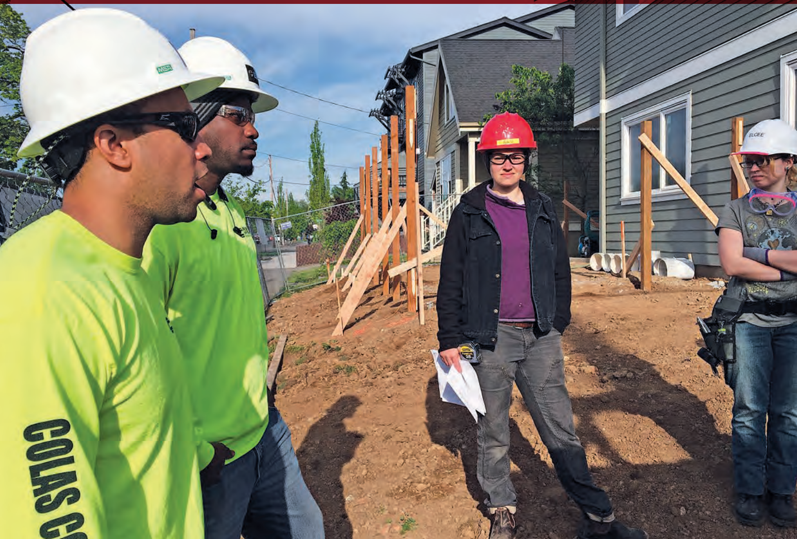
6th and Ainsworth Townhomes under construction (PCRI).
